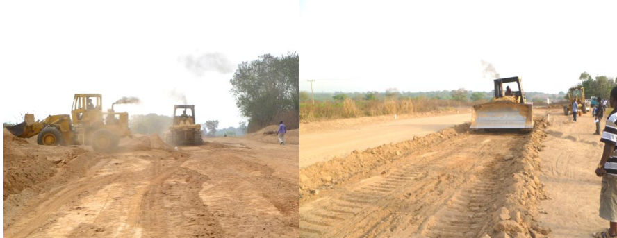
Tractor fumes and dust discharged into the air during clearing (Authors field work, 2014)
