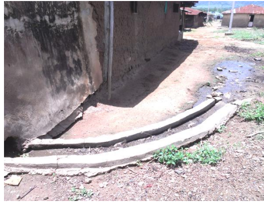
Drainage pattern in Okin village (Authors' field work, 2014)
