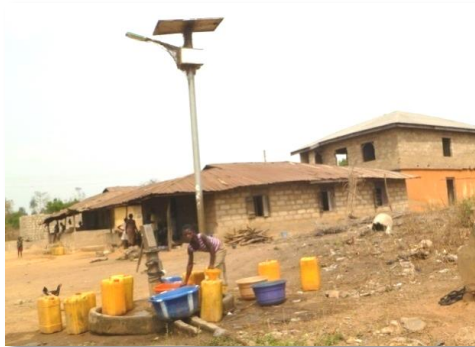
The marked hand-pump, solar system and buildings in Okin village (Authors’ field work, 2014)
